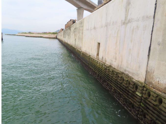
General View of Vertical Eco-shoreline
