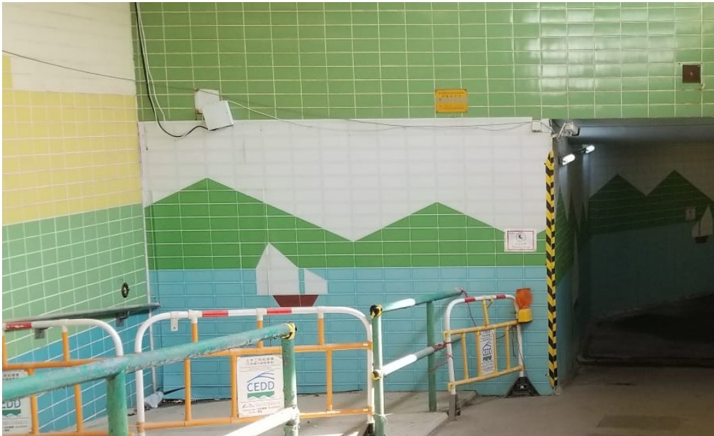
Photo 3 – Erection of site hoardings in unobtrusive colours
